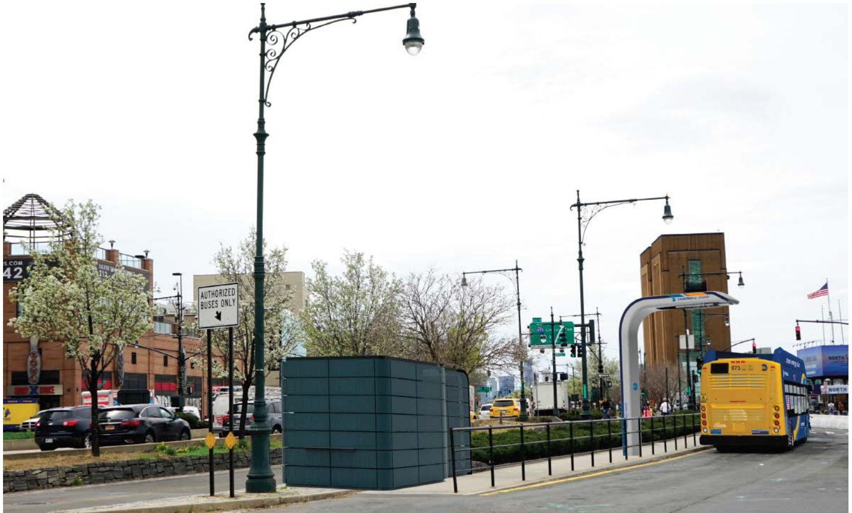
Terminal for M42 and M50 , West 43 rd Street, Manhattan, Circle Line
