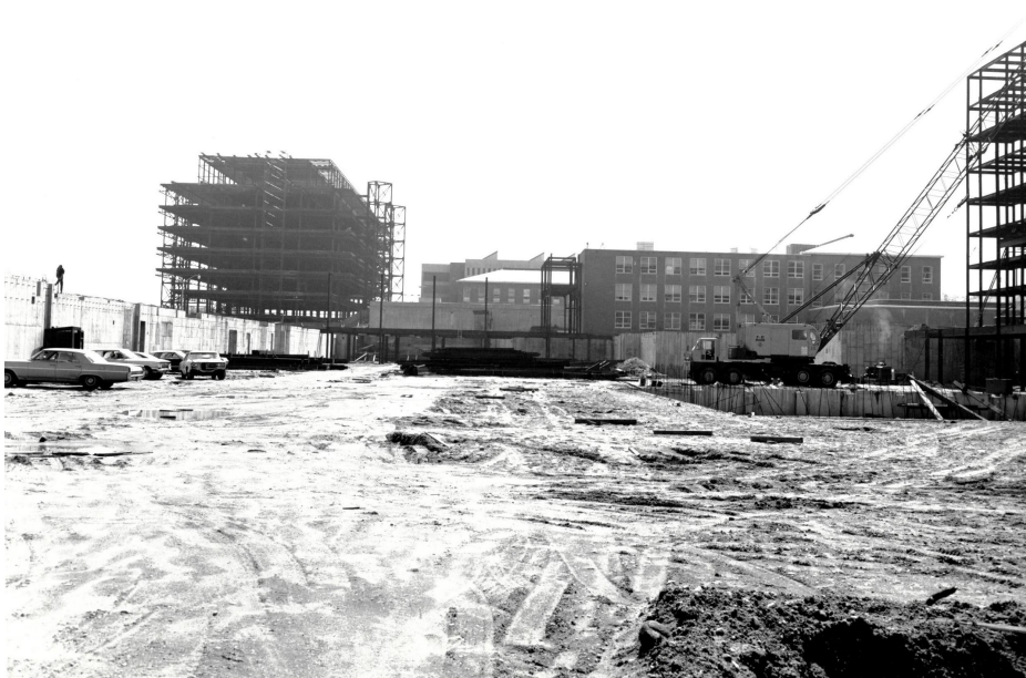
Left: Chemistry building
